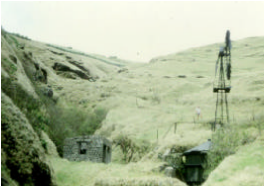
The Windmill used to pump water through the Tunnel from the wells in Breakneck Valley, photographed in 1979. Today, the vanes have fallen off and the structure is rusting away.
