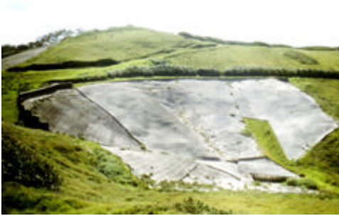
Breakneck Valley rain catchments, these are no longer used.
